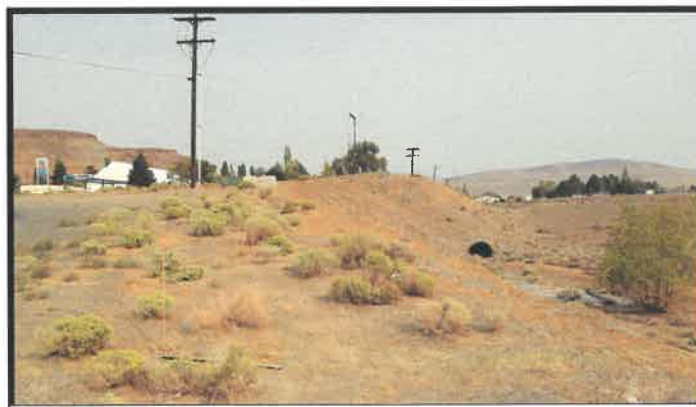
End of existing 72" CMP Culvert. Looking North.
