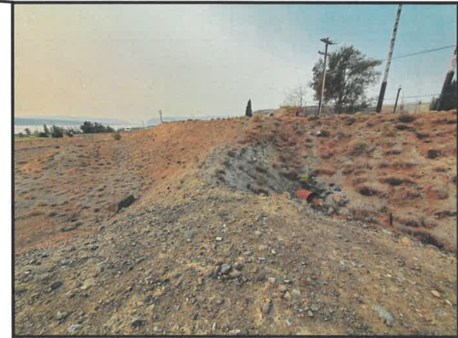
Upstream side of existing 72" CMP culvert. Looking south.
