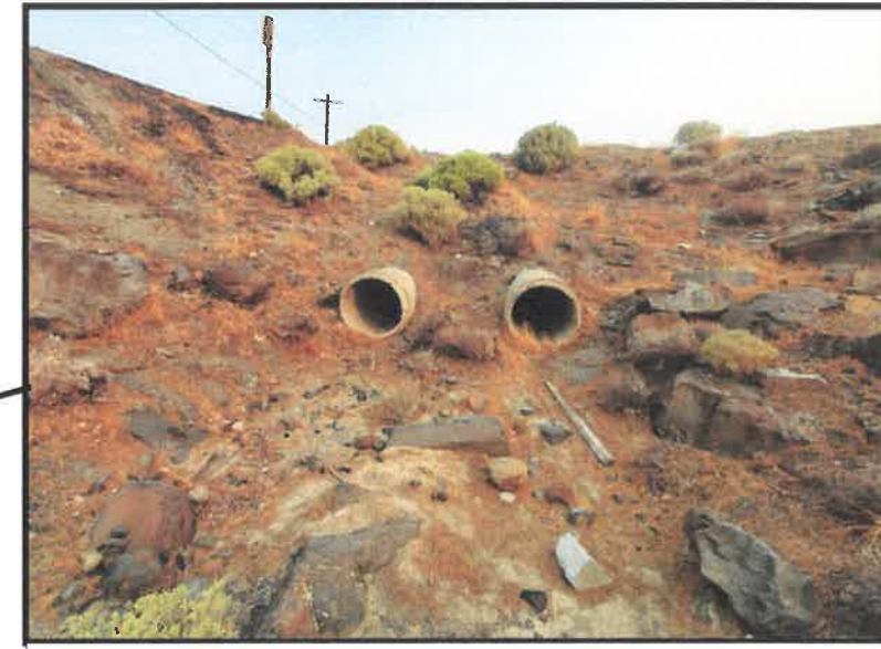
Downstream end of existing 36" culverts. Looking towards Wayne Street.
