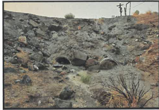
Existing 36" culverts. Upstream (northside) of Wayne Road
